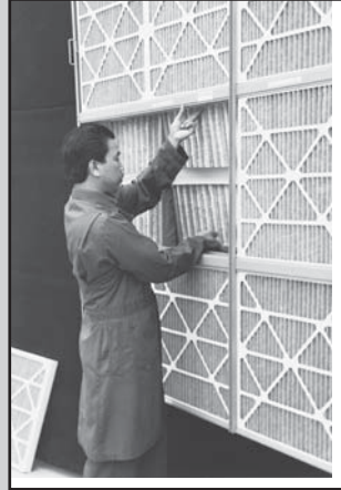
Installing filters and prefilters
